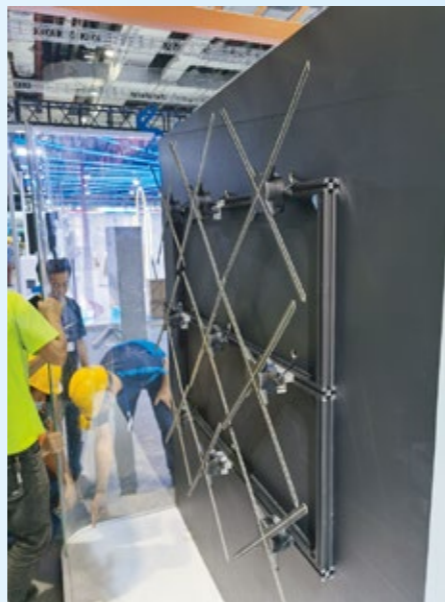
On-site installation effect
